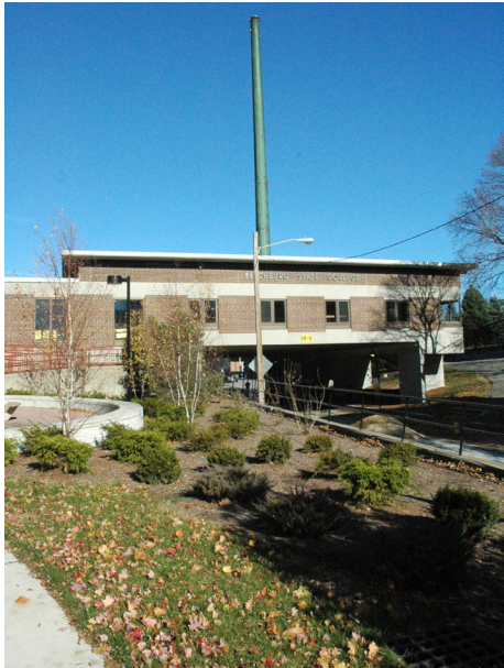
Holmes Dining Hall Bridging North Street
