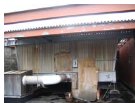
Original cooling tower ACM panels?
