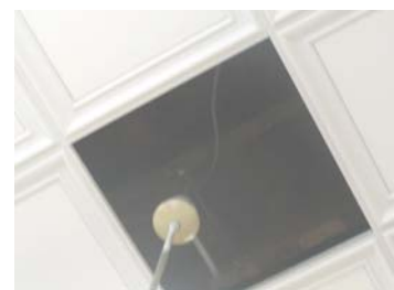
New hung ceiling. Note timber.
