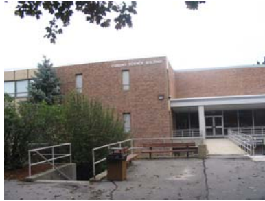
Front entry, with shared pedestrian bridge with Sanders.
