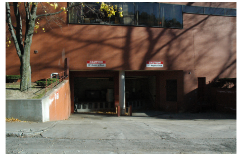
The Hammond Center Loading Docks on North Street Reinforce A Service-Oriented Character of that Corridor
