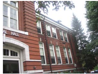
Note Vent. Shafts to roof, and UV wall louvers.
