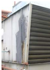
Large patch on cooling tower.
