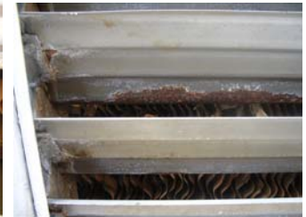
Corroded slats.
