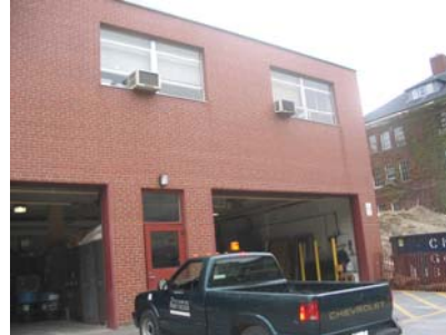
Window AC units.
