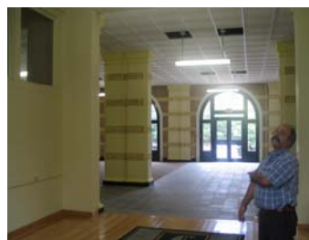
Lobby, early done with Renov.
