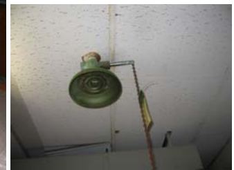
untempered emergency eye wash and showers. Outdated and considered unsafe.
