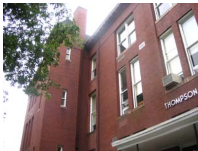
Window AC units.
