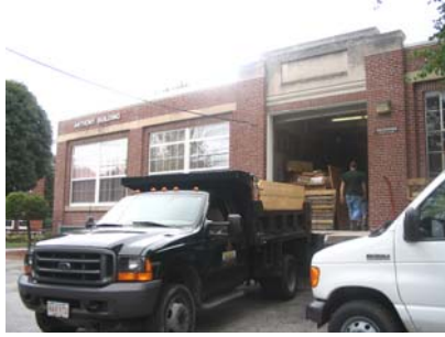
Front & Loading dock.
