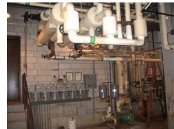
MER with hung heat exchangers.
