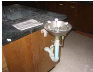
untempered emergency eye wash and showers. Outdated and considered unsafe.
