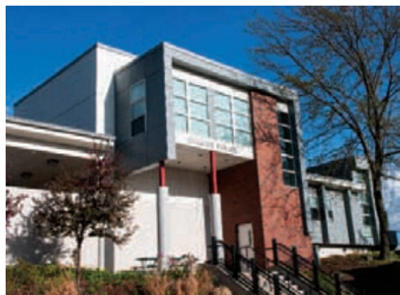
The Campus Police station, built between Clinton and North streets, has improved safety for the university and the neighborhood.
