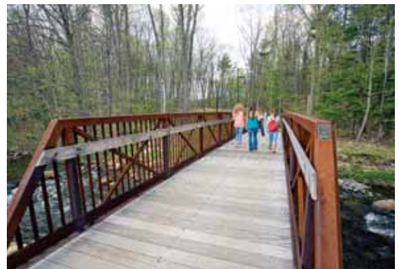
A pedestrian bridge and paved walkway link the Civic Center to the athletic fields.
